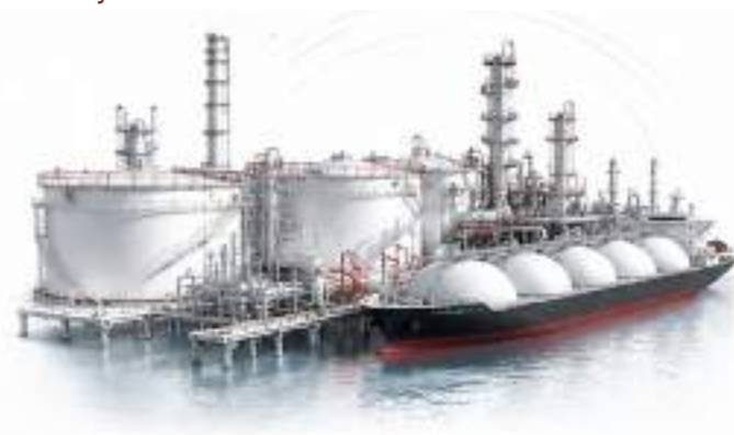
Oil and gas terminals
